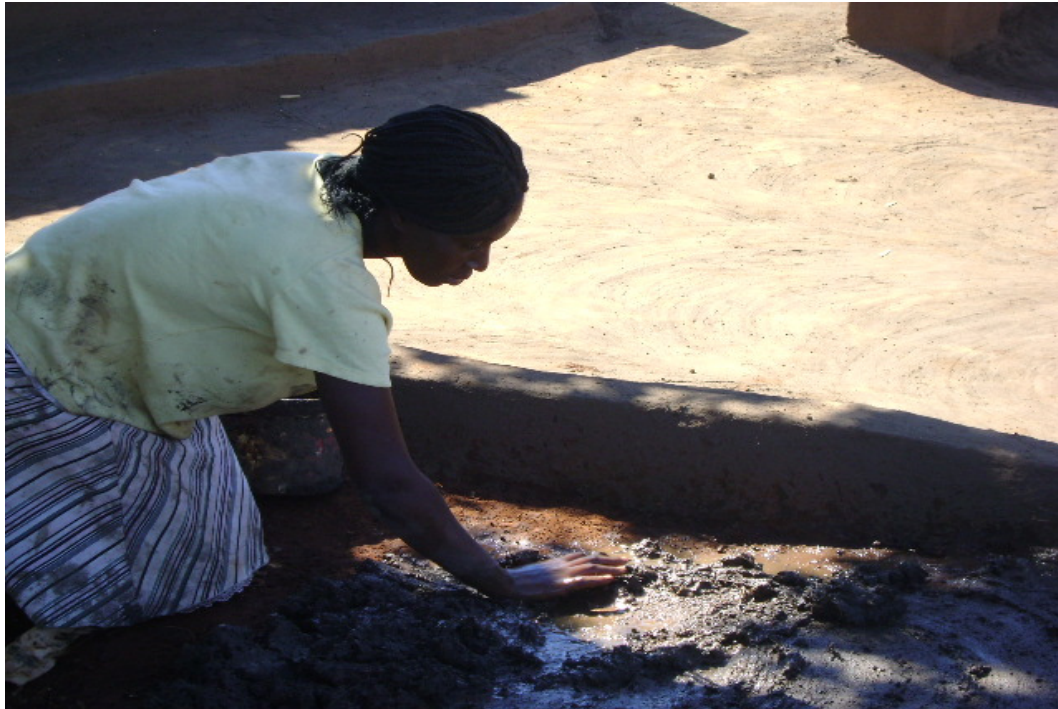
One of the women is seen polishing the floor with cow dug.
