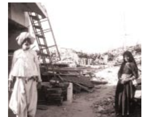
Destruction caused by the rapid onset of the Gujarat earthquake on 26th January 2001
