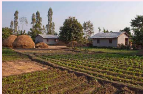
Two newly built concrete homes in Bardiya District, Nepal.
